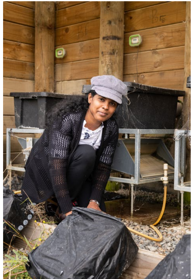
PhD student Sarmini Maheswaran checking drainage flow meters in a drainage pit at Massey University
